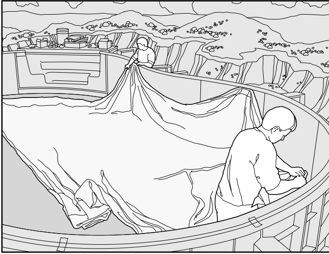
2. Unfold the liner with the arrows pointing at the shallow end corners. Note plywood and 2x4 with strip to hold liner during install.
